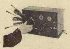
Observe the change in pitch of a C.W: note when the hand is withdrawn from the dial.
