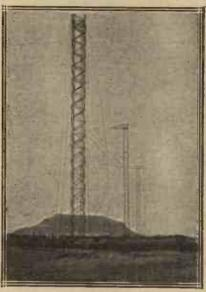
The great beam station near Poona, in India, is making rapid progress. The five masts are each to be 297 feet high, and they are being sent out from England in sections. They are 12 feet square and the cross arms are 20 feet long.
