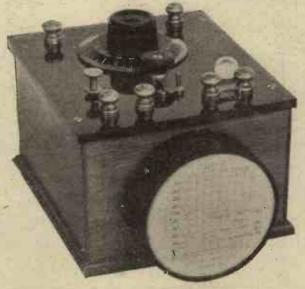
condenser is employed, the capacity is 300 micro-microfarads, and when both are used together the capacity is brought up to a total of 800 micro-microfarads. The advantage of this is, it is stated, that the small condenser can be used for tuning over the higher broadcast-frequency range when fine control is more important, and that on the lower frequencies a larger band can be covered by using both condensers in parallel.
