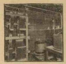
The oscillatory circuits of one of the intermediate amplification stages at Rugby.
