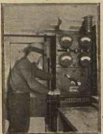
Wireless will play an important part in the operations of the U.S. Navy polar expedition under Commander Byrd. The S.S. "Chantier," a lake steamer of 3,000 tons, will form the base of the expedition, part of the power panels of her transmitter being seen here.
