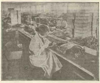
Assembling telephones at the B.T.H. works. Our photograph show the closing of the clips on the leather head-bands.
