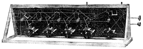
Fig. 4.—Rear view of the supersonic receiver with local oscillator detached.
