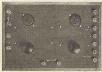
Fig. 2.—Anti-vibratory valve sockets are used.
