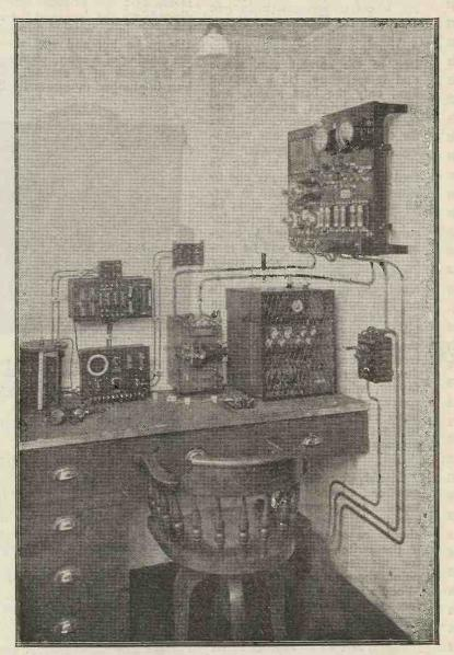
Our photograph shows a standard Marconi transmitter and receiver for shipboard use. Apparatus of this type may be seen at the Palace of Engineering, Wembley.
