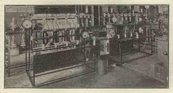
Water-cooled valves in use at the high-power broadcasting station at Chelmsford (5XX).
