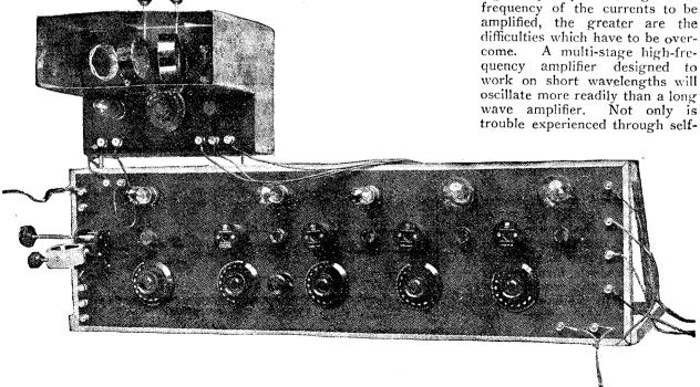
Fig. 1.—An experimental supersonic heterodyne receiver used by the author in his experiments. The local oscillator is contained in the metal screened box on top of the instrument.
