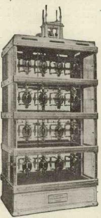
The Marconi "Value Pillar"-A method of assembling transmitting values which is both neat and safe.
