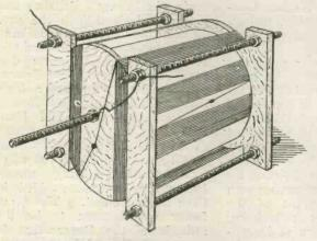
Fig. 1.—The completed variometer.
