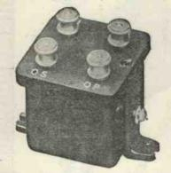
Fullers United Electric Co.'s inter-valve transformer.
