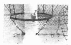
**Fig. 2.** The base of the fibre-glass supporting pole of the mast aerial is also the feed-through insulator. The ring at the bottom is a rain-cone.
