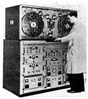
ic tape record was first demonstrated to members of the Press. 55 This was a two track stereo recording initially mastered at 15 i.p.s. and then duplicated down to 7.5 i.p.s. for domestic consumption.
