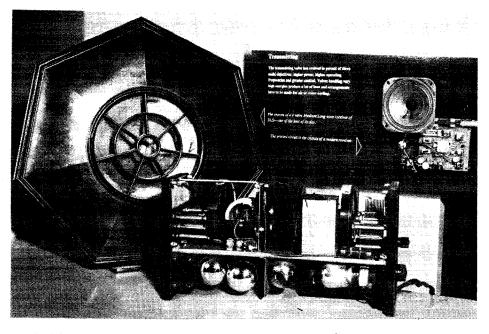
On the left the chassis of a 1923 medium- and long-wave receiver and on the right its present-day equivalent. These are two Philips radio receivers on show in a display covering the story of radio at the newly opened extension of the IBA's Broadcasting Gallery, Brompton Road, London.
