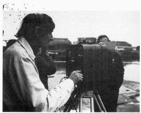
Engineer seen operating the remote unit of a Tellurometer microwave measuring system during winch-out of "Graythorp One", the world's largest oil rig, on the first stage of its 250-mile journey to BP's Forties Field.
