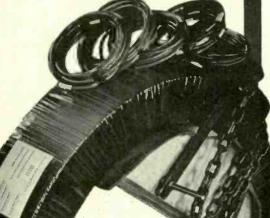
Telcon Mumetal used in a large bushing current transformer, manufactured by Smith Hobson Ltd., which was one of several for the Niagara Falls Generating Station.
