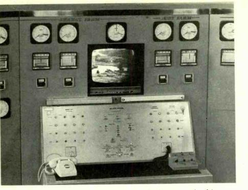
Telemetry and television supervisory control position at the Horning master station of the East Anglian Water Company showing monitor picture as received over the low bandwidth cable link.
