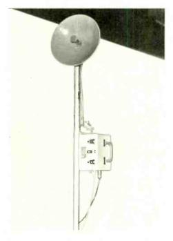
Receiving paraboloid, with translator on the mast, for the 12GHz service.
