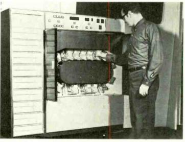
RCA video tape cartridge recorder/player with 18 cartridges, each providing 1-3 minutes' playing time.
