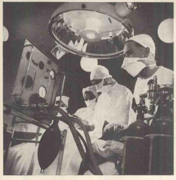
The Electronic Lung A member of the Pye Instrument Group W. Watson & Sons Ltd. has produced an electronic lung which is capable of replacing an iron lung. The Barnet Ventilator, as the instrument is called, is transistorised and is easily portable in cases of emergency. It is shown here in its application in an operating theatre for the administration of anæsthetics.
