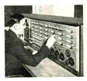
AUTOMATIC SWITCHING. Sound broadcast programmes for the B.B.C.'s West Region transmitters are switched to their destinations by a system something like an automatic telephone exchange. It is operated by a single engineer at this control desk, which is the "nerve centre" of a new control room recently installed at the West Region headquarters in Bristol.
