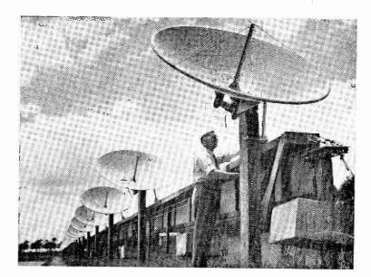
**C** OR studying localized sources of radiation on the sun, an Australian radio astronomer, W. N. Christiansen,\* has designed a highly directional aerial system with a beam width of only one-twentieth of a degree. This extremely narrow beam is necessary because of the small angular width and spacing of the radio sources. The angular width of the sun itself is only about half a degree, so obviously the beam must be
