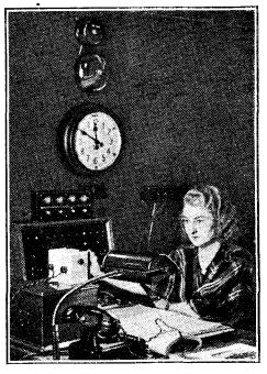
A POLISH TIME SIGNAL. A two-bell system worked in conjunction with the minute and second hands of the clock is radiated by the Poznan station.
