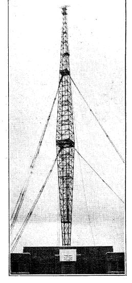
The last word in broadcasting aerials is this vertical type in which the mast is itself used as an aerial. Efficiency can be raised to as high as 80 per cent.
