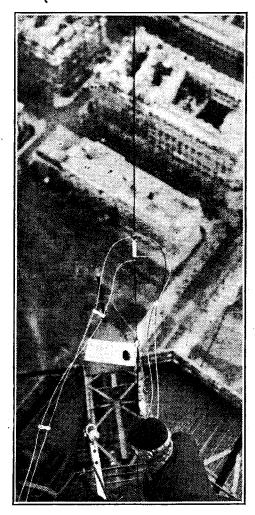
Fig. 1.—The feeder system to one of the aerials on the summit of the Eiffel Tower is clearly shown in this illustration.
