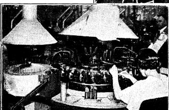
as glass tubing which is fed into a vertical carrier above one of the rotary glass-working machines. The tube is first cut to the required length, then heated and flanged, and the top half flattened ready for sealing in the wires.
