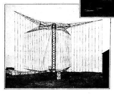
The addition to a beam aerial of a reflector, as shown in this photograph, considerably enhances its directional properties.
