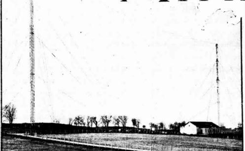
High power alone does not account for the excellence of the Athlone transmissions. The station is situated on an ideal site 300 feet above sea level, and the masts are 330 feet high.
