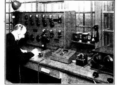
AN AERIAL TELEGRAPH OFFICE. The Marconi directional receiver installed in the control tower of the new Manchester Air Port at Barton Moss. Telegraph and telephone messages are picked up from aircraft in flight.
