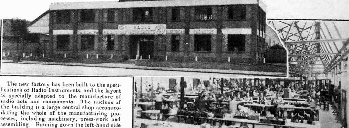
dating the whole of the manufacturing processes, including machinery, press-work and assembling. Running down the left-hand side are the stores for raw materials and finished products with doors opening on the outside to a concrete roadway for loading and unloading vans and lorries. The works manager's
