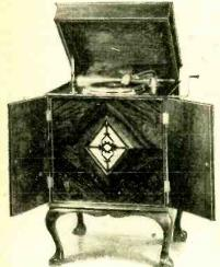
The Panatrope electrically reproducing gramophone. The valves are mains-fed as is also the field magnet of the moving coil loud speaker.
