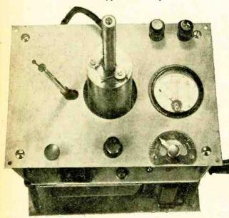
Plan view with paper-carrying cylinder withdrawn. Space is left on the top panel for accommodating other forms of recording gear than the electrolytic stylus. The stylus is stationary.
