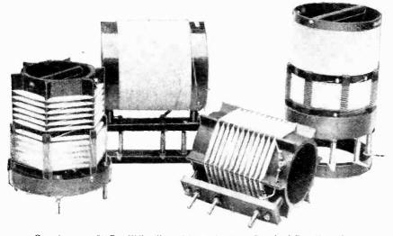
Complete set of "Berchit" coils and bases for the "Standard Four" receiver. A 20
