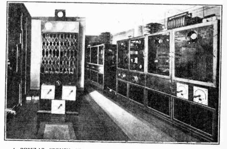
A POPULAR FRENCH STATION. The transmitting room at Radio Toulouse, showing the 5-kilowatt transmitter which is capable of working up to an aerial power of 9 kilowatts. Radio Toulouse celebrates its third birthday on April 15th.
