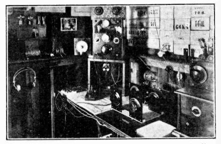
A NOTTINGHAM AMATEUR TRANSMITTER 2HD, owned and operated by Mr. Aubrey Harper at Cropwell Bishop, Notlingham, has been in touch with most European countries on wavelengths of 23 and 45 metres, and with an input of 4.5 watts. The transmitter shown is of the Hartley type. The receiver is a Reinartz.
