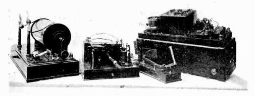
TRANSMITTING AND RECEIVING APPARATUS AS USED ON THE "LAKE CHAMPLAIN."
