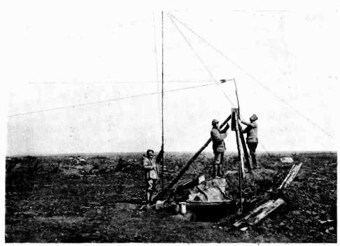
[French Official Photograph. ARRANGING THE "LEAD-IN" OF A WIRELESS AERIAL ON THE FRENCH FRONT.
