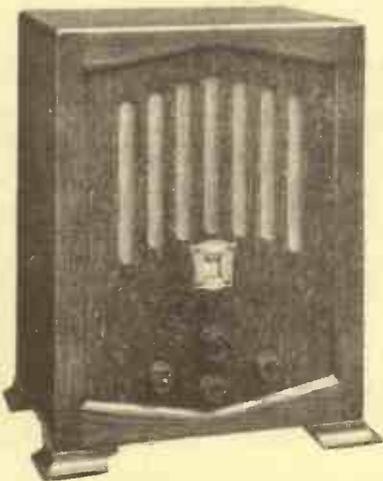
The Kolster Brandes Electric Kobra, a three-valver with a detector and two low-frequency stages
