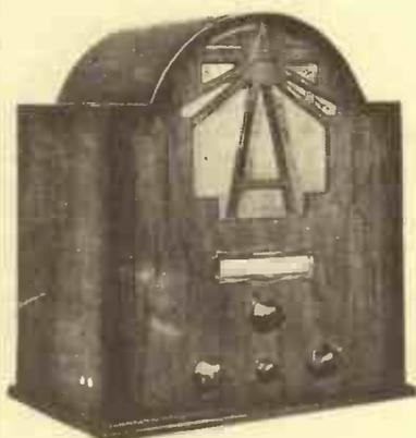
A set from the Sovereign range, The Doric. It is a battery three-valver with moving-coil reproducer
