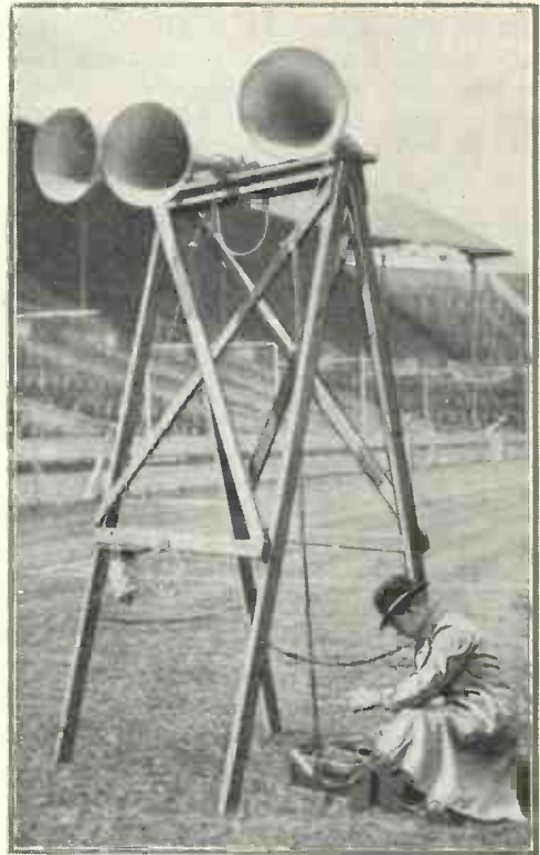
PREPARING TO MAKE SOME NOISE! A public-address engineer testing the loud-speaker installation at Wembley Stadium in preparation for a cup final. Moving coil units are used
