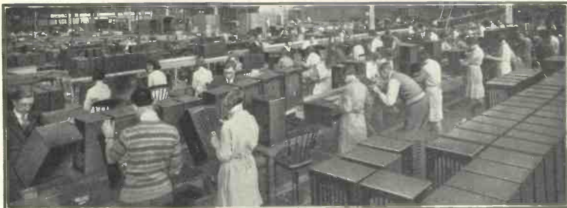
A BUSY SCENE IN A MASS-PRODUCTION FACTORY Assembling receivers in the well-equipped Kolster-Brandes factory at Sidcup, Kent. Many well-known sets have been produced at this works
