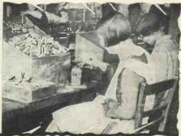
Making the zinc cells for Siemens high-tension batteries
