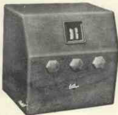
The Marconiphone model 39 is available as a mains-operated set. It uses a screened-grid valve, and the price is £21
