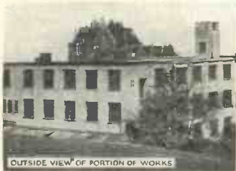
OUTSIDE VIEW OF PORTION OF WORKS
