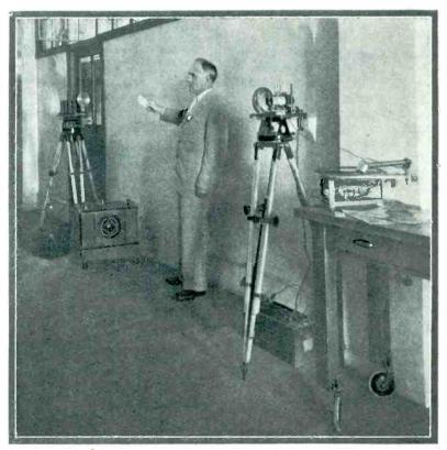
John Bellamy Taylor holding his hand in the path of the music-carrying light beam. To the left is the receiving apparatus and loud-speaker; to the right the electric equipment. By varying the amount of light permitted to pass, the operator can control the intensity of the reproduced sounds
