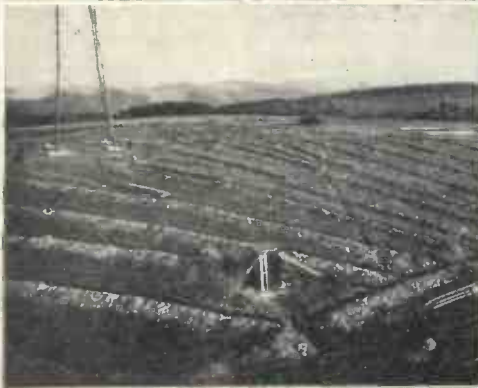
Trenches for the elaborate "earthing" system used at Langenberg.
