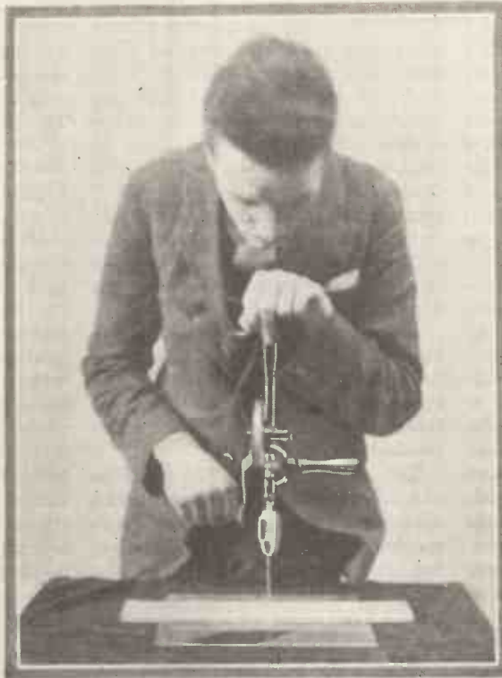
Drilling a Glass Panel.
