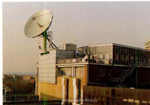
A 9-metre dish installed at Television Centre in 1991, for reception and transmission of satellite signals
