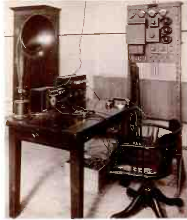
Control position instrument room GEC works, Witton, Birmingham
