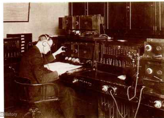
The Birmingham Control Room, 1931
