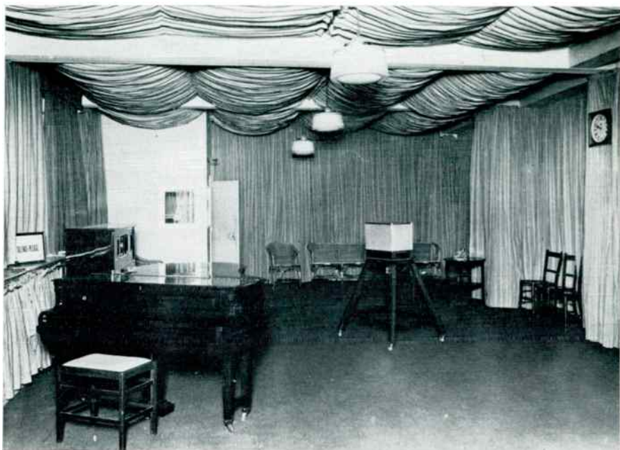
7 'Drama' studio at Savoy Hill, 1928: A late example of a heavily draped studio using a 'meatsafe' microphone
