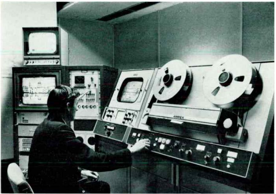
22 Videotape machine: A high proportion of programmes are pre-recorded on tape and edited before transmission
