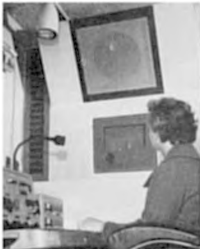
BBC Studio Manager checking quality during a record programme. This loudspeaker was specially designed to fit into a corner recess. The most suitable distance for monitoring in the studio is between three and six feet from the speaker
