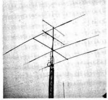
Typical amateur radio station lattice tower with 3-element tri-band h.f. beam plus v.h.f. arrays mounted above. Suitable Buccaneer applications on this installation are a balun connection to  $50\Omega$  coaxial cable and rotator control cables
