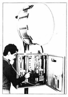
GEC 19GHz narrowband digital microwave radio equipment
