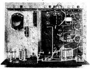
Top view of one of the famous series of receivers designed by S.T., the ST300 of 1932.
