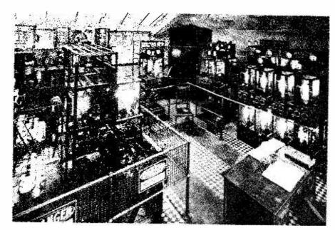
A first glance at the transmitter hall of 2LO gives the impression of many mighty kilowatts but in fact it was only 1.5kW. On the right are the early audio stages and modulator with the master oscillator in the centre background. The power supply with its transformers and valve rectifiers is on the left.
