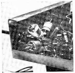
The arrangement of the concentric trimmers around the programme switch.
