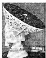
Backed by considerable experience in the design of steerable aerials, AEI's Electronics Group has designed the new aerial to be steered with a pointing accuracy of two minutes of arc, in winds of up to 45m.p.h. The drive motors which will steer the aerial's 82ft. dish-which together with the rest of the moving structure will weigh approximately 300 tonswill be supplied by AEI's Motor and Control Gear Division,
