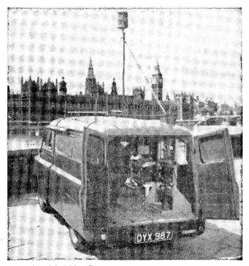
A member of the LCC staff is seen here switching on an EMI tape recorder in a van at an Albert Embankment site, in London, to record sample noise levels (see "Recording Noise").
