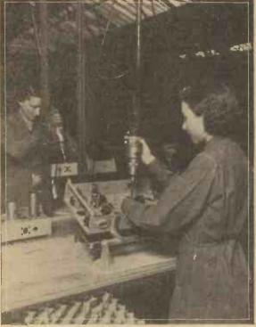
Automatic screwdrivers and spanners, suspended on overhead springs, make component-mounting a swift and simple operation at the Ekco works.
