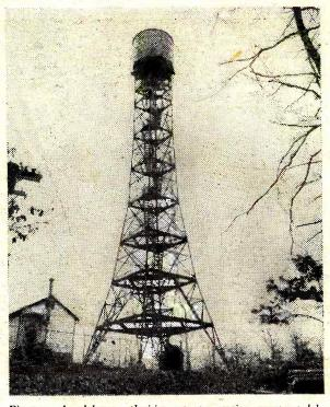
Fig. 20.—An elaborate television repeater station, constructed by R. C. A. Communications to relay programmes from Long Island to New York. The picture signal is sont by frequency modulation in this equipment.
