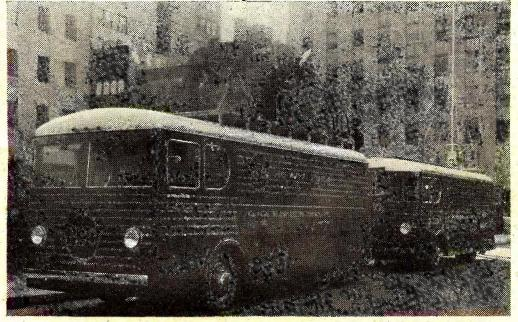
Fig. 17.—The N.B.C. mobile television vans. The microphone is mounted in a parabolic reflector to pick up the sound at a distance, while the camera is fitted with a telescopic lens. The transmitter can is at the rear.
