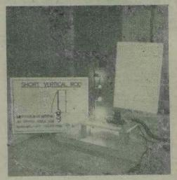
Fig. 2.-Current distribution in short vertical aerial.
