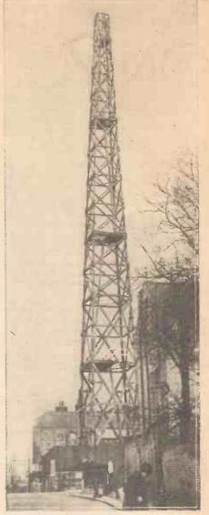
A new television mast 150 ft. in height is now being erected for the outside broadcasts of television. The existing aerial at Alexandra Palace interferes with other programmes. This one, on the top of Highgate Hill, will be well away from any interference.
