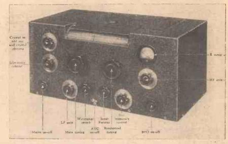
The controls of the Eddystone E.C.R. Two pointers are provided on the dial so that bandspreading may be accurately carried out.
