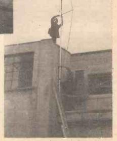
The upper mast being fixed in position on the tower.
