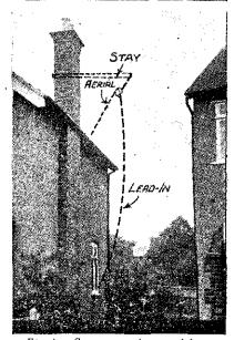
Fig. 4.—Supporting the aerial from a short stay fixed to a chimney.
