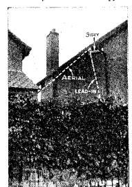
Fig. 3.—A stay can be used for keeping the lead-in away from the house wall.
