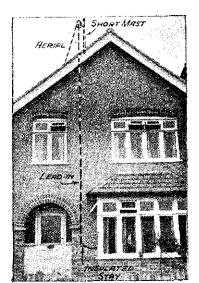
Fig. 5.—A short mast can be used where the aerial is taken over the top of roof.
