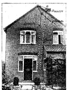
Fig. 1.—Method of attaching aerial to the point of the roof.
