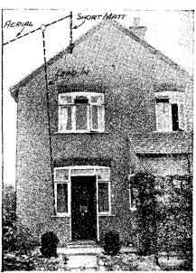
Fig. 2.—Using a short mast for anchoring the house end of aerial.
