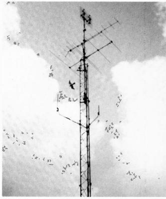
Roger's DX aerial mast complete with Les Wallen 27 and 49MHz aerials and full-size plastic decoy falcon to the rear of the Band I array.
