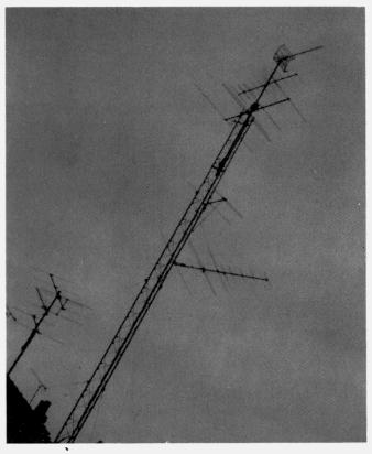
New aerials and mast in my back garden. The guy wires are at 20 and 30 feet. (No, the mast isn't really at the angle shown here!)
