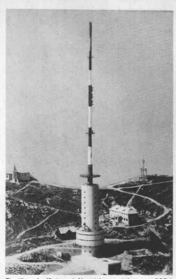
The Klagenfurt/Dobratsch (Austria) transmitting mast. ORF-1 is transmitted on ch. E10 at 160kW, ORF-2 on ch. E24 at 1,250kW. The site is at 2,115 metres while the mast is 155 metres high. Photograph courtesy ORF, Vienna.
