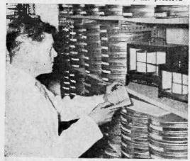
Checking thermograph and hygrograph in the vaults.
