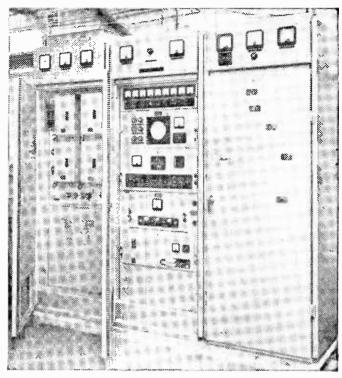
The Royal Board of Swedish Telecommunications has placed another order for television and sound broadcasting transmitters with Marconi's Wireless Telegraph Company Limited. This picture shows a BD 366C 5 kW Band III vision transmitter, 14 of which are included in the order.
